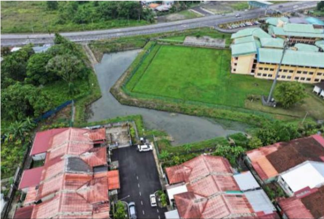
Dry Detention Pond at SK Muara Tuang, Samarahan
