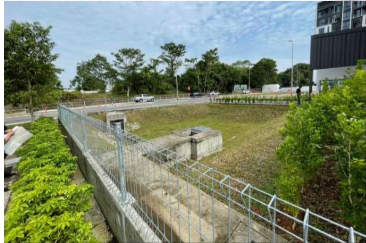
Dry Detention Pond at Dayak Chamber Of Commerce And Industry, Jalan Simpang Tiga
